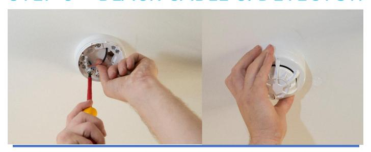
Blue Light Safety will install an Apollo Orbis multicriteria detector as the trigger mechanism for the system, the black cable (supplied by Blue Light) must be installed by yourselves before installation day.
