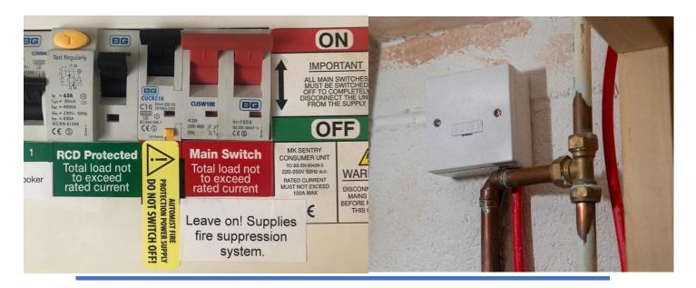
No more than 1m from the water supply there should be <u>1x non-switched</u> <u>fused spur fitted with a 13amp fuse</u>. This must be run in <u>FP200 cable (1.5 or 2.5).</u>
