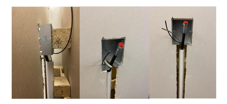
The high pressure hoses and cables (supplied by Blue Light) must <u>enter from the bottom</u> <u>of the backbox</u> and must be fitted so that it <u>can be retracted from the backbox</u> by around 100mm for fitting of the heads and to service the unit in future.
