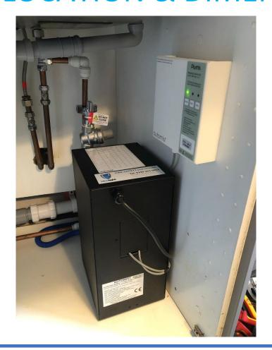
The Automist pump is approx. 385mm (height), by 216mm (depth) by 181mm (width).
